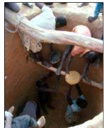
construction of a well
